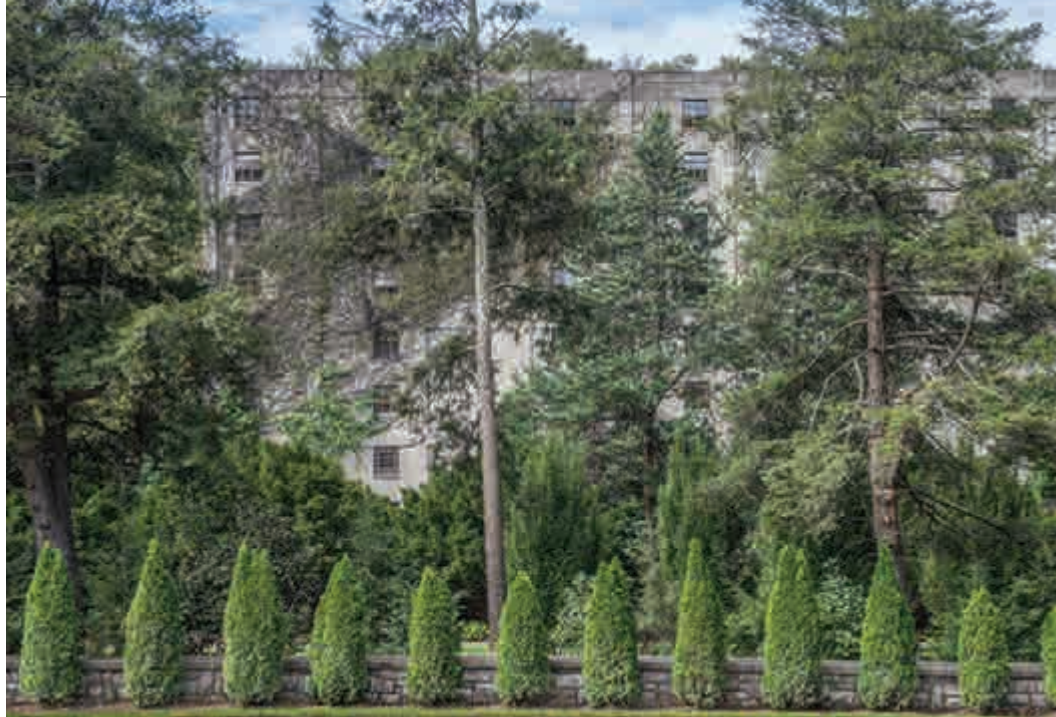
Castle & Key's largest aging warehouse can hold 65,000 barrels.
