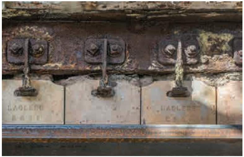
Original ironwork references the distillery's past.
